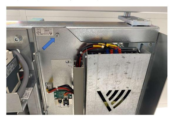
20. Re-mount the left-hand cover of the ceiling wagon using the five screws.
