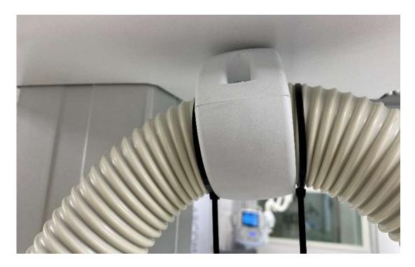
8. Release and remove the two Torx T20 screws for the cable holder and hang down the cable.
