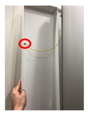
**1.4.9** It is now possible to follow the cable routing all the way from Bucky to Canon powerbox. Disconnect it in Canon powerbox end and pull it out towards the bucky, using a separate wire or cable attached to the charger cable.
