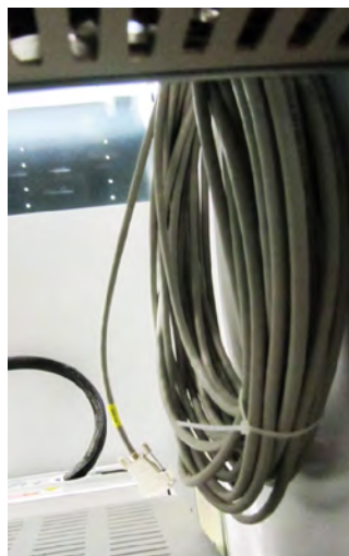
Gen. Console cable is hanging, rolled together, inside the cabinet.
