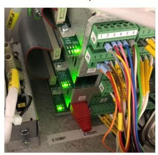
CB01 LEDS: D1=OFF, D2=OFF, D3=FLASHING, D4=ON
