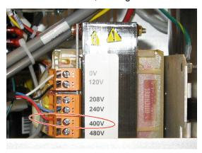
Fig. 4-36 Connection 400V
