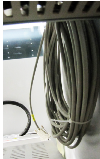
Cable 732 091-00 is hanging, rolled together, inside the cabinet.
