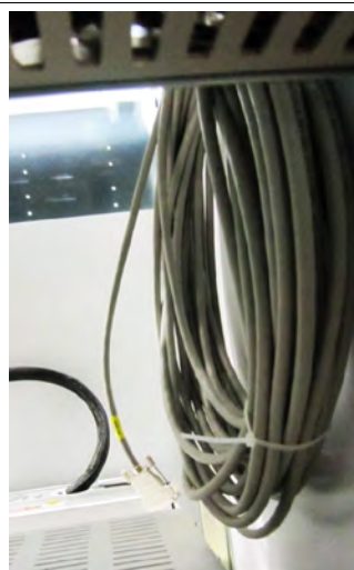
Cable 732 091-00 is hanging, rolled together, inside the cabinet.
