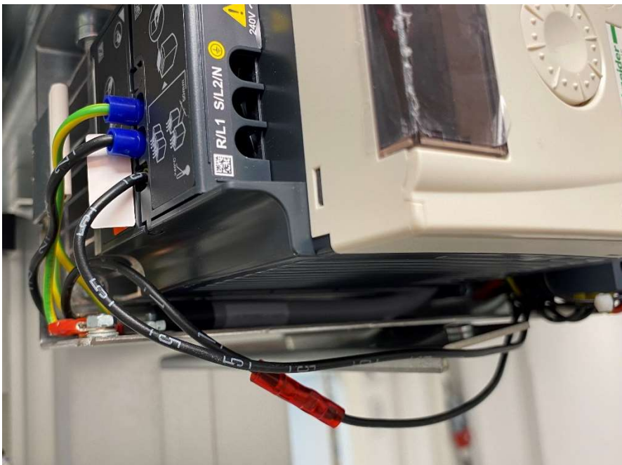
Column motor connections to 1.2FC01 (wire 4-5).
